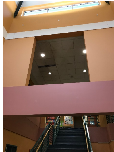
View of cut-out window looking up the stairs
